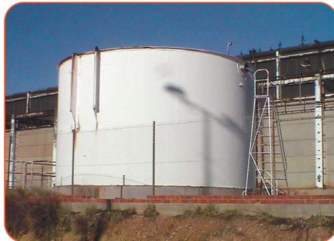
Mercury Sludge Tank.
