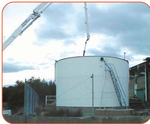
Encapsulation of the mercury sludge.
