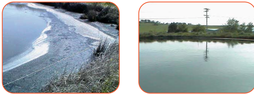
Figure 8 – Leachate pond – Before treatment (left); after treatment (right)
