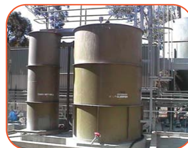
The plant's bioreactor and secondary clarifier.
