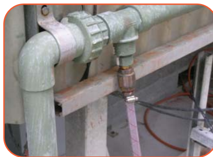
Dosing point for ViroPhos™ reagent A (above) and ViroPhos™ reagent B (below).
