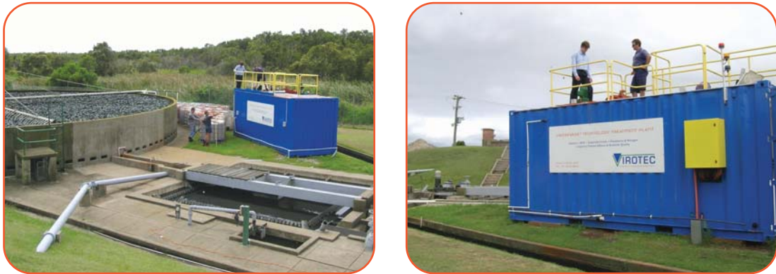
Fig 2. The ViroSewage™ Technology dosing plant being installed at Evans Head.
