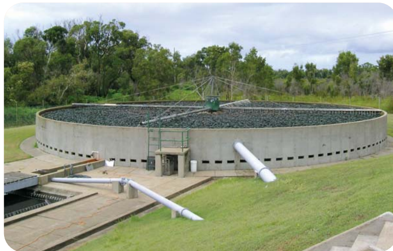
Fig 1. The Southern trickling filter at Evans Head sewage treatment plant.
