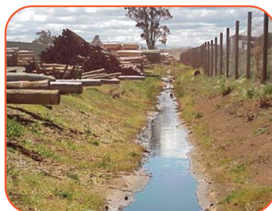
Figure 3 - The stormwater drain leading from the timber storage area to leachate pond.
