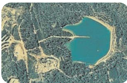
An aerial shot of the Tailings Dam.
