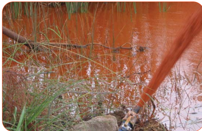
Dosing of ViroBond™ reagent into leachate pond, suspended heavy metals rapidly settle to the bottom following treatment
