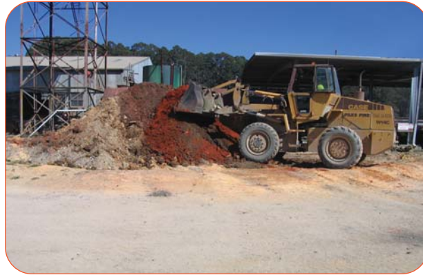
Treatment was applied using a loader
