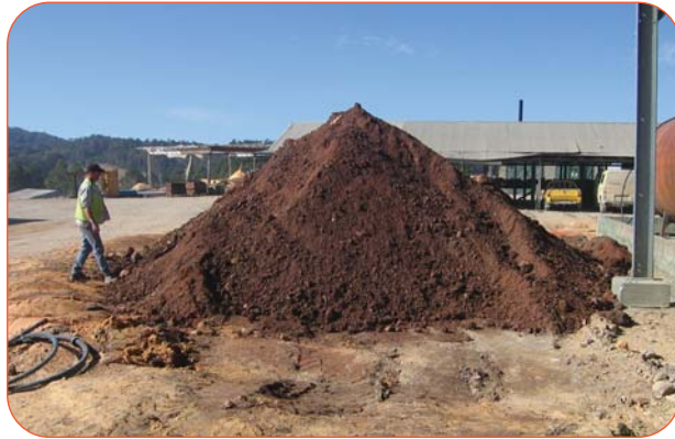
Treated CCA stockpile after ViroFlow™ Treatment
