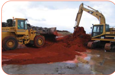
Figure 2 - Treatment was applied using an excavator and loader
