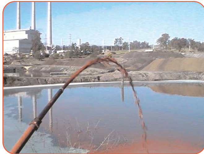
Leachate Pond No.3 During Treatment with ViroFlow™ Reagent A.
