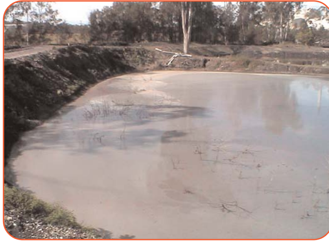
Leachate Pond No.3 before treatment.
