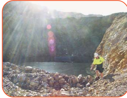
Contaminated water generated in the quarry pit was pumped to the Western Holding Dam.
