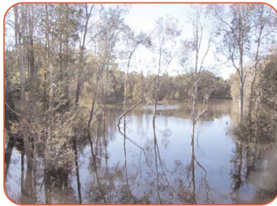
The Western Holding Dam located in a pre-existing wetland area.
