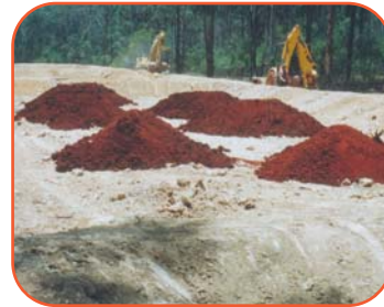
Photos showing sulphidic, acid generating rock and in-situ soil remediation in progress.
