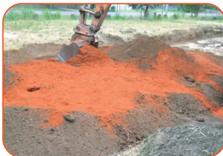
ViroBind™ reagent being mixed into contaminated soil.
