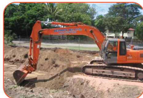
ViroBind™ reagent being mixed into contaminated soil.
