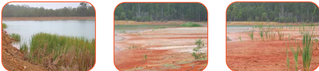
Figure 3. After the treatment and discharge of the tailings dam water, wetland plants have been able to colonise the exposed tailings beach. Before treatment using Acid B™ and Terra B™ no vegetation was able to colonise the exposed tailings or exposed dam walls.
