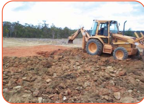
Figure 8 (Left): Terra B™ being mixed into the zinc-enriched tailings with the backhoe. Figure 9 (Right): The fully remediated Zn-enriched tailings plot at Rossarden prior to revegetation with poa grass seedlings.
