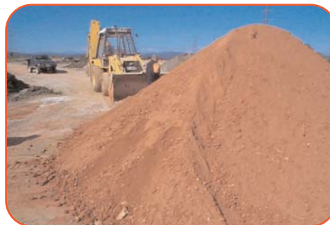
Figure 6: 26 tonnes of stockpiled Terra B™ reagent at the materials handling staging area in Tasmania.
