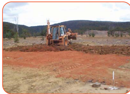
Figure 7: Terra B™ being spread onto the zinc-enriched tailings with the backhoe.
