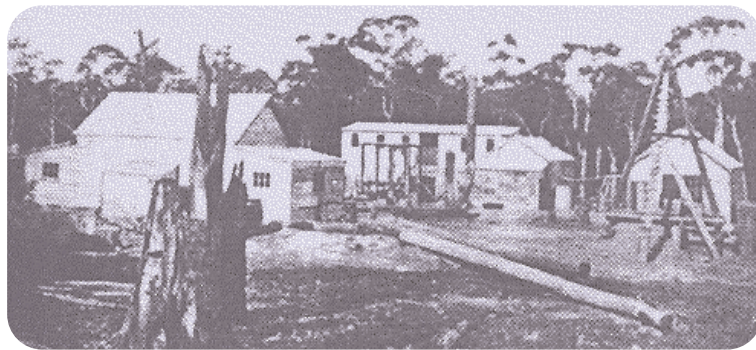
Figure 1: A 1931 view of the Rossarden mine site with, from left to right, the blacksmith's building, the mill building and the main shaft.
