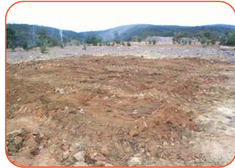
Figure 8 (Left): Terra B™ being mixed into the zinc-enriched tailings with the backhoe. Figure 9 (Right): The fully remediated Zn-enriched tailings plot at Rossarden prior to revegetation with poa grass seedlings.
