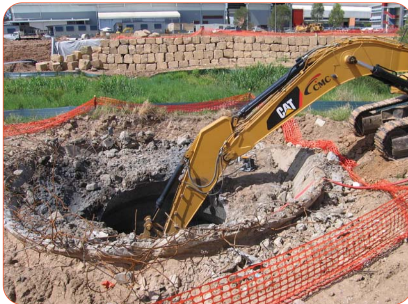
Figure 2 - Excavation of sludge from underground tank
