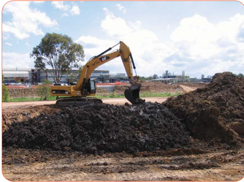
Figure 3 - Treatment of sludge and contaminated soil in the “Designated Treatment Area”
