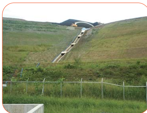
Figure 5: Photograph showing the source of the leachate from the highway (top centre) and the diversion channel (centre) used to divert leachate to the ViroMine™ Technology filter system (bottom left).
