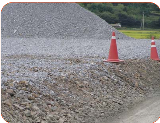
Figure 1: Highway construction at Cheongju City (left) and sample of the pyritic rock responsible for generating sulphuric acid and metal contaminated leachate (right).
