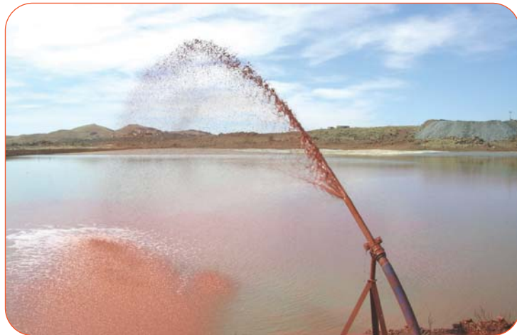
Figure 3: Acid B™ reagent slurry being applied to the tailings dam.
