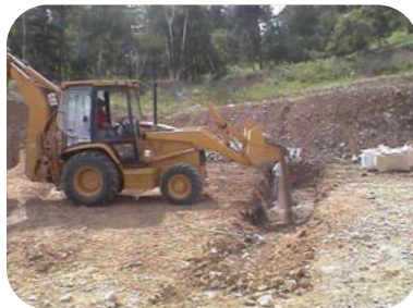
Preparing the Permeable Reactive Barrier Trench.
