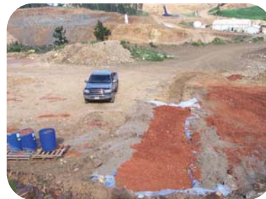
Preparing the Permeable Reactive Barrier Trench.
