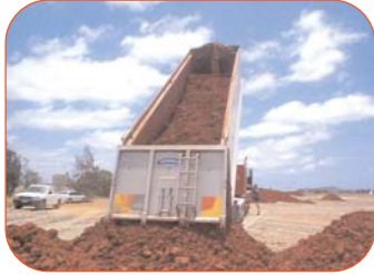
Application of ViroSoil™ Technology reagent into Marine Sediments.
