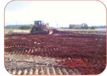
Application of ViroSoil™ Technology reagent into Marine Sediments.
