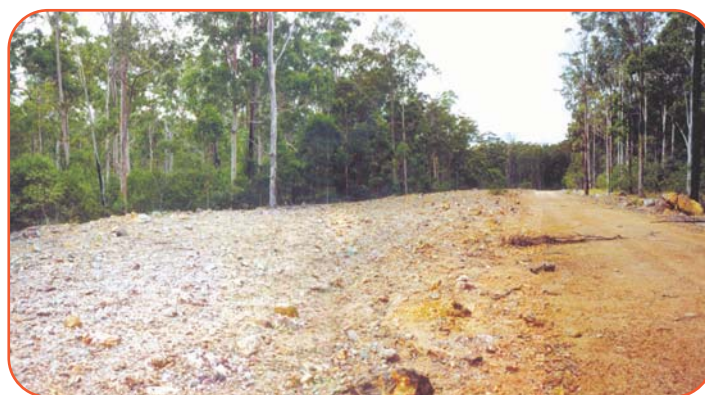
Figure 1. The study site three years ago showing the failure of previous liming for remediation ten years before.
