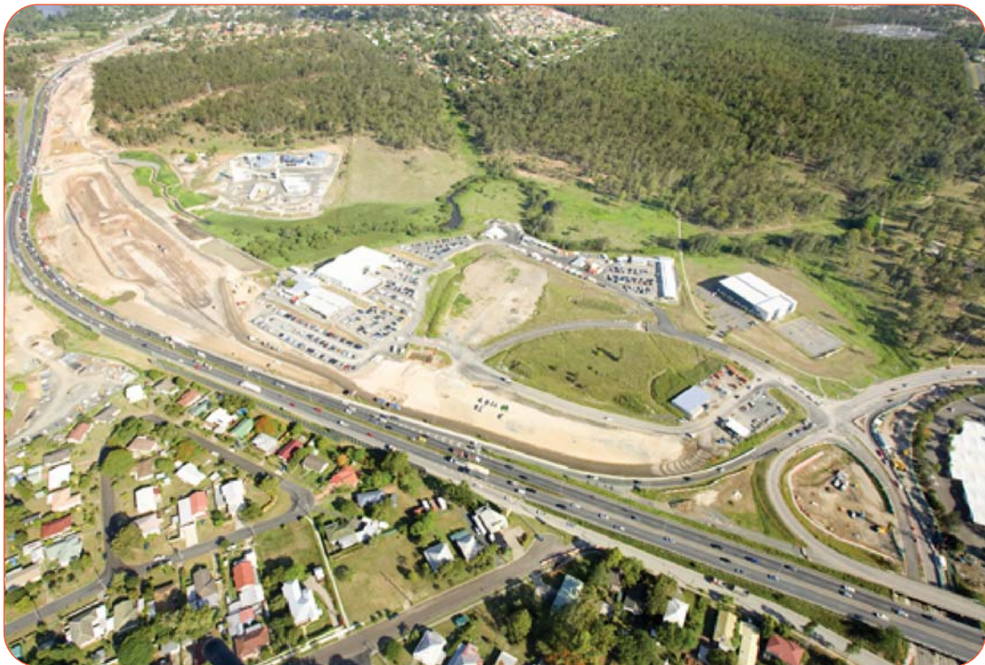
Figure 1 - An aerial view of the Dinmore to Goodna motorway upgrade
