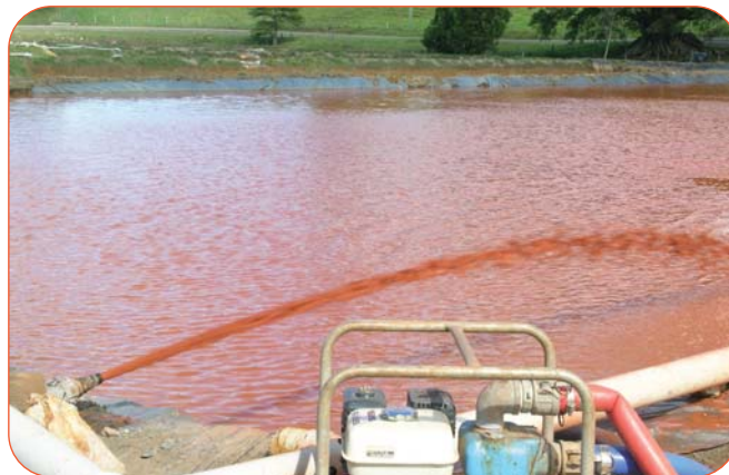
Figure 3: ElectroBind™ reagent being sprayed over the dam surface.
