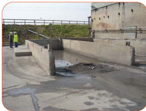
Figure 2: Two of the collection pits where the metal-contaminated site run-off is collected by mechanical sweepers prior to pumping to the holding lagoon.
